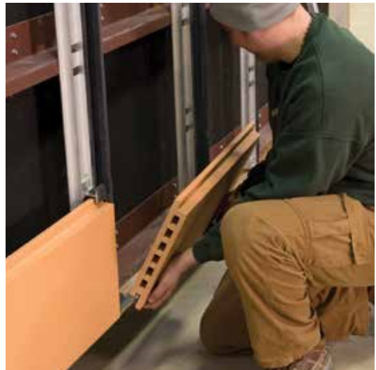
Install TerraClad™ panels
