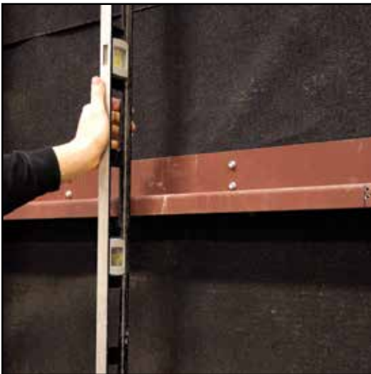
Prepare site and install track
